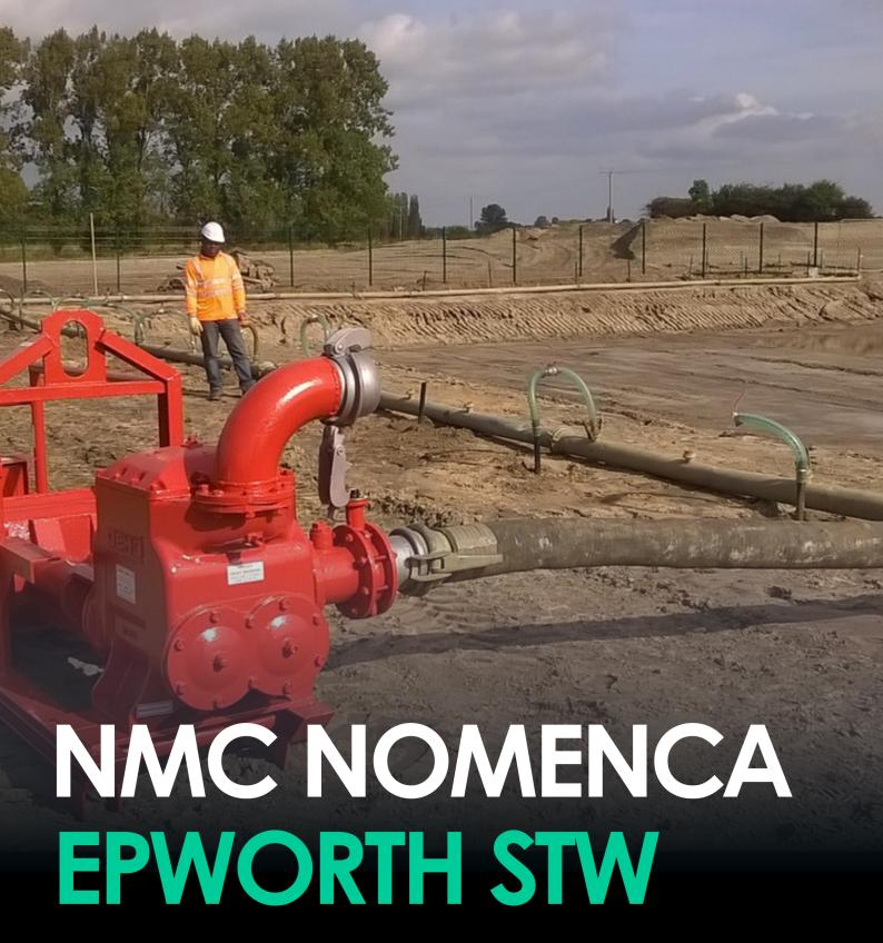
Vacuum wellpoint dewatering of 4no Final Settlement Tanks with settlement assessment and monitoring
