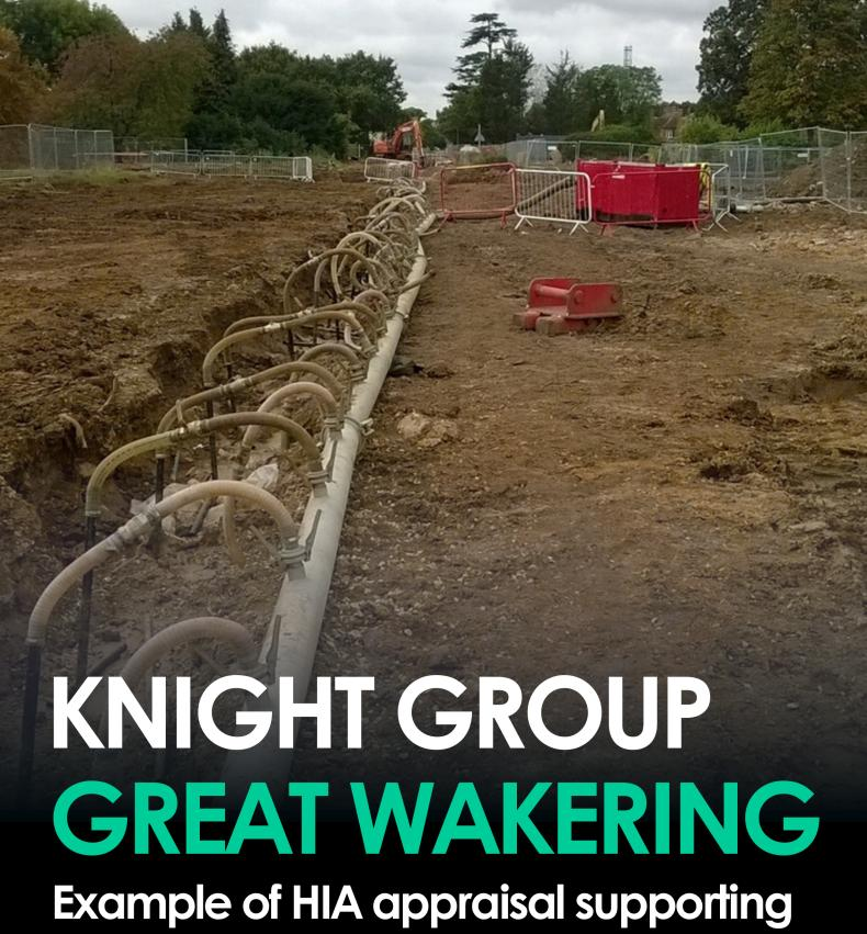
Example of HIA appraisal supporting an application for a groundwater abstraction licence for a dewatering system at a housing development
